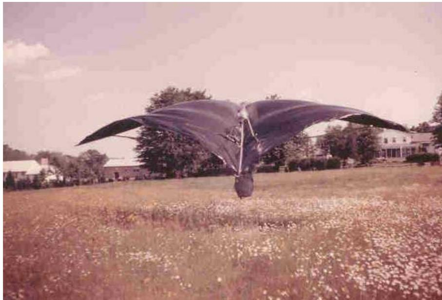
Foot launched powered parawing around 1963, 7 hp West Bend driving a 3 foot dia. glass over balsa propeller. Main structure is 6061-T6 aluminum tubing, 4 mil
